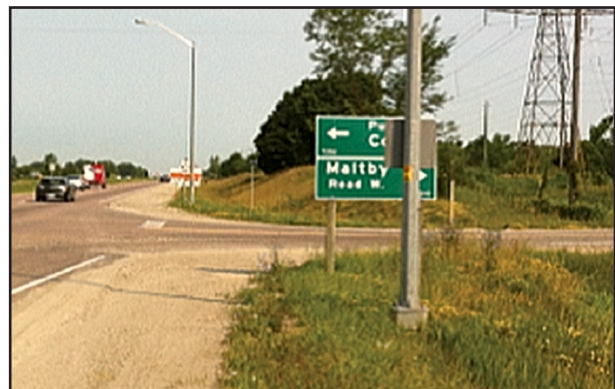
The smaller square sign in this picture attached to the pole cannot be read from any direction. It has been installed in a poor location facing the information sign.
